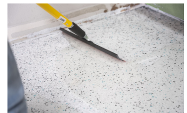
Grout Coat Squeegee
