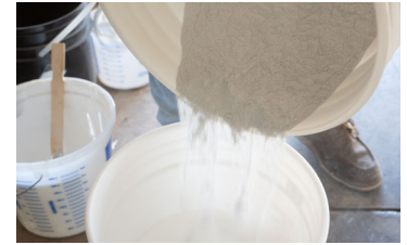
Mixing PozzoFill™ w/ Epoxy
